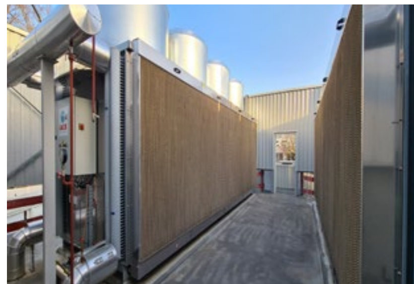
The CNRS is attempting to find sustainable solutions to renovate and maintain its research buildings and equipment. Here, we see the cooling system for the Jean Zay supercomputer. The machine's heat will be recovered and fed into the Paris-Saclay urban campus's heat and cold exchange network.
